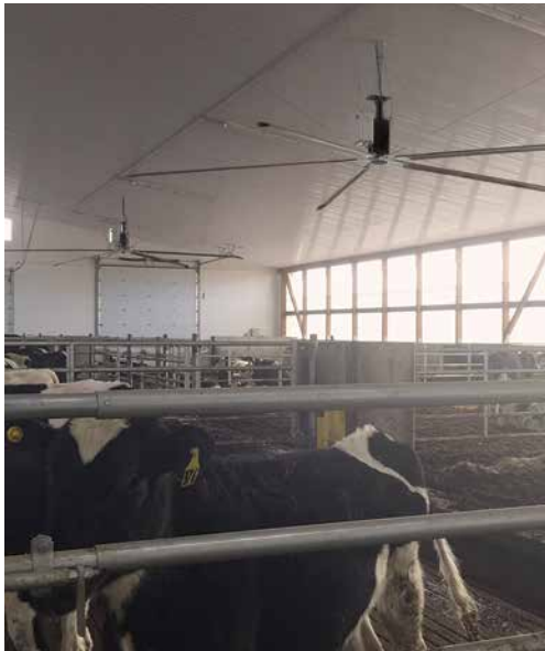
Series of Industrial Class fans used in dairy barn for ventilation and destratification.
