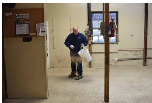
Color chips in a five color blend were broadcast into the wet basecoat to create a finished, high-end terrazzo look.
