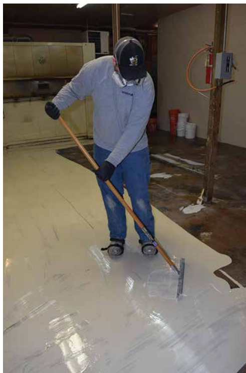
A beige pigmented ultra-low VOC polyaspartic basecoat was applied at 15 mils thickness. The basecoat was squeegeed then backrolled.
