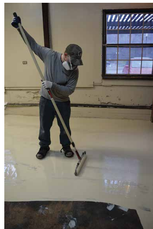
A beige pigmented ultra-low VOC polyaspartic basecoat was applied at 15 mils thickness. The basecoat was squeegeed then backrolled.
