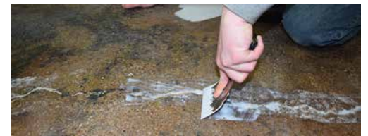
Application of an epoxy mortar to cracks and large defects.
