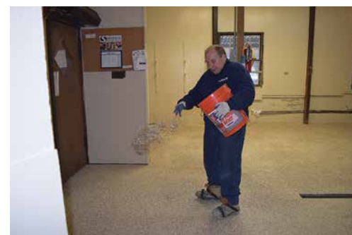
Color chips in a five color blend were broadcast into the wet basecoat to create a finished, high-end terrazzo look.
